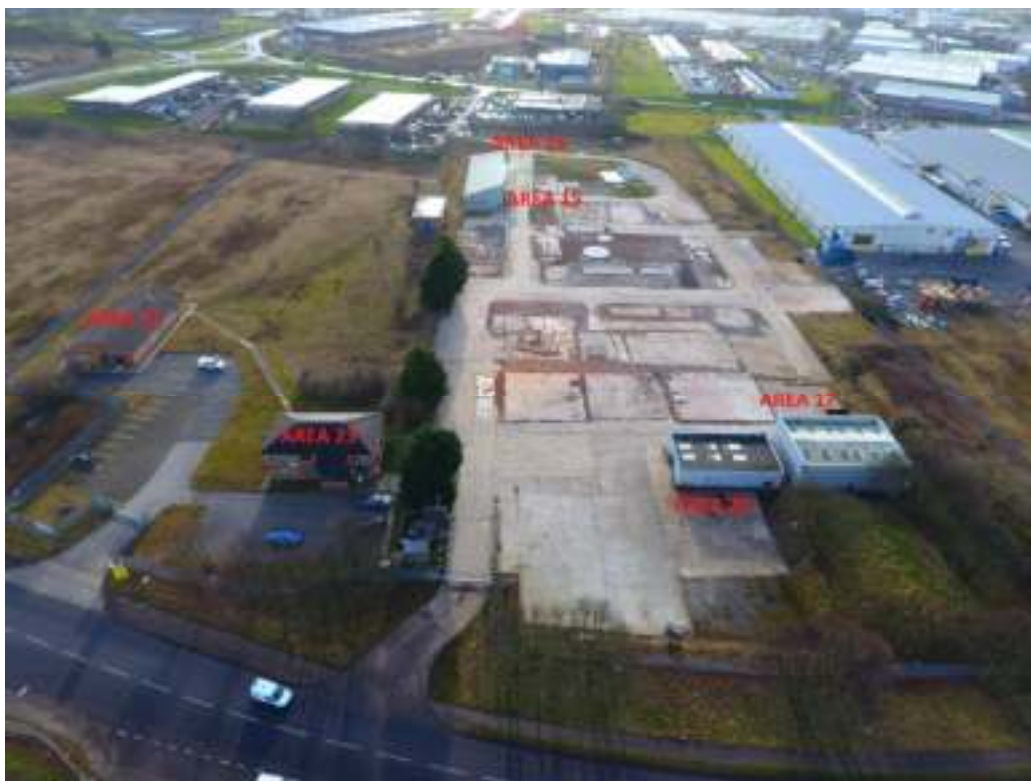
(Photograph of cleared site – February 2020)
